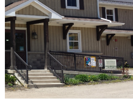
Exterior accessibility improvements
